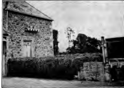
FIG. 232. — Manure pile on the island of Jersey with cistern below to collect liquid manure.
